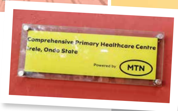
Above-Left, Centre and Right: The Health Centre now has clean running water at all times as a result of the solar-powered borehole and an alternative power battery system installed by the Foundation.
